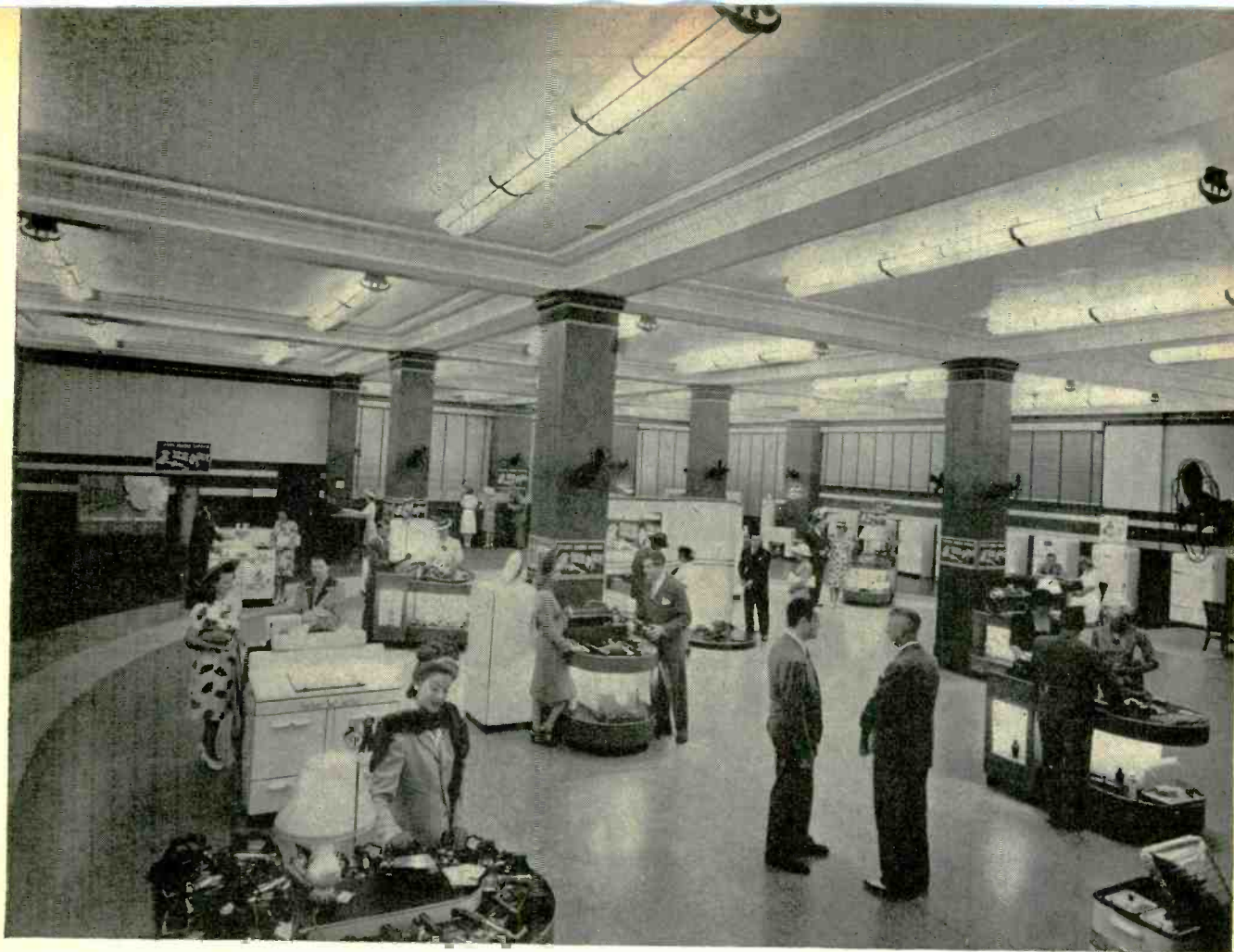
Above: good levels of general store lighting by means of standard fluorescent lamps and fixtures. Customers are encouraged to circulate throughout store, look at more merchandise displays. Island displays indirectly lighted or with portable lamps. Across, top: Fluorescent fixtures are easily cleaned without special tools. For installation data, see spacing chart on page 36.
